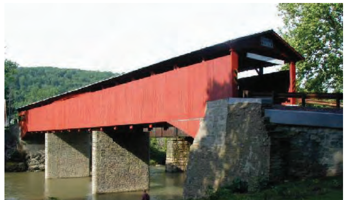
The Rupert Bridge was originally built in 1847 and rehabilitated in 2000-2001
