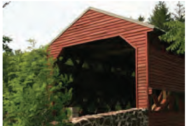
The Sachs Covered Bridge was used by both Union and Confederate troops during the Civil War
