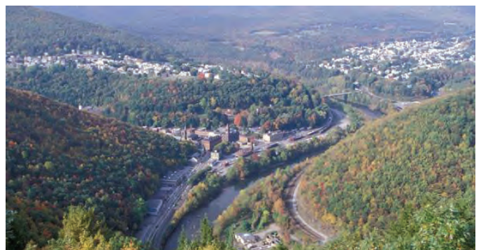
The Jim Thorpe Bridge is programmed to be replaced in the first four years of the TYP
