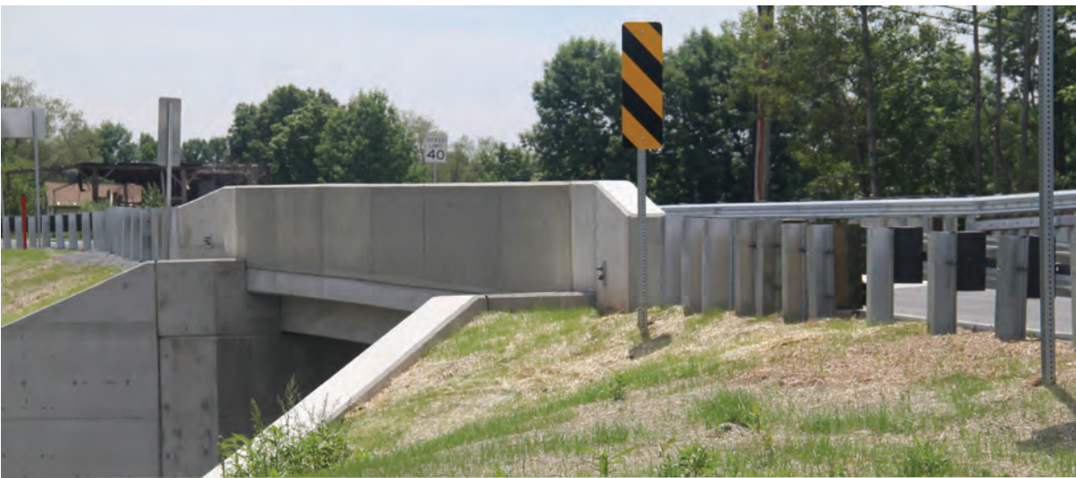
The Cherry Ridge Bridge Project in Wayne County
