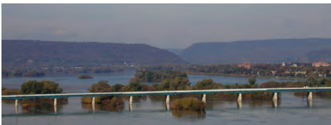
The Harvey Taylor Bridge over the Susquehanna River
